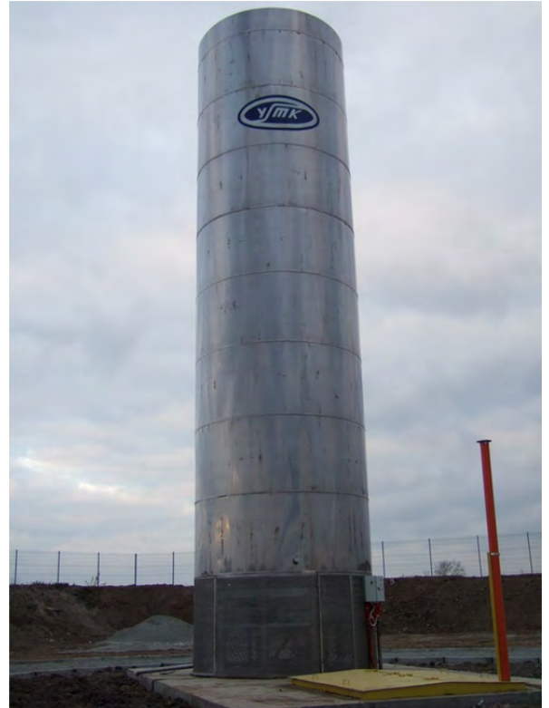
Bio Gas Burner (25 MW) with combustion chamber for the Flare
