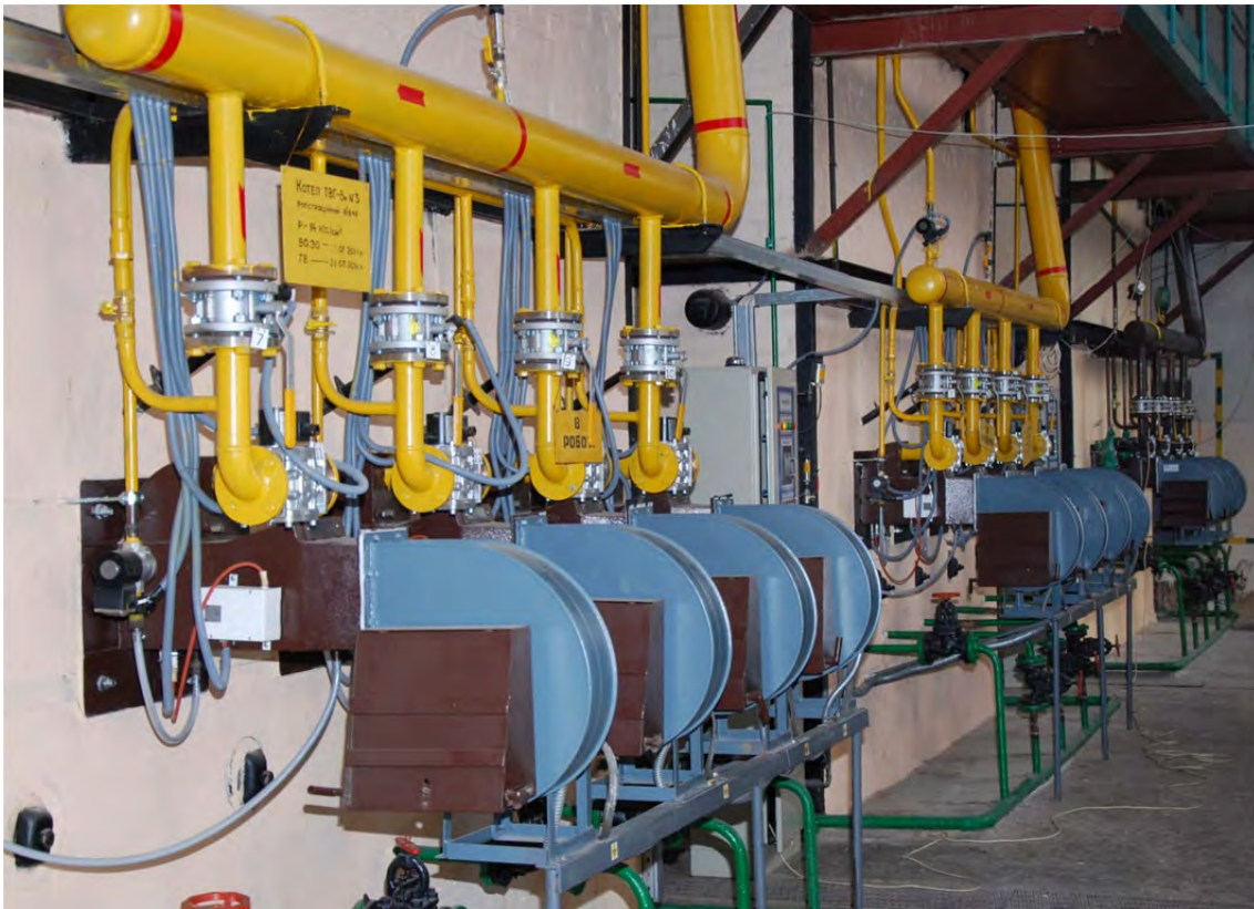
Water-heaters with MD Gas Burners
