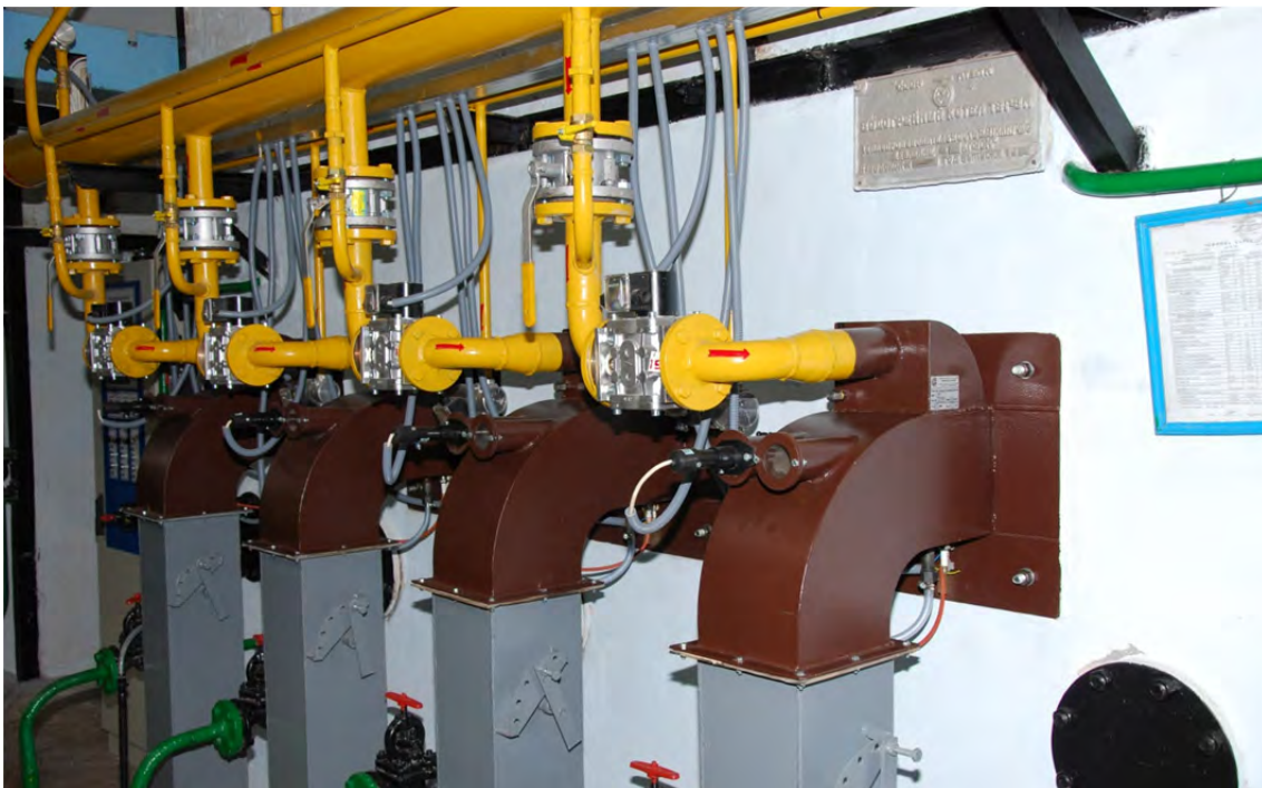
Water-heaters with MD Gas Burners
