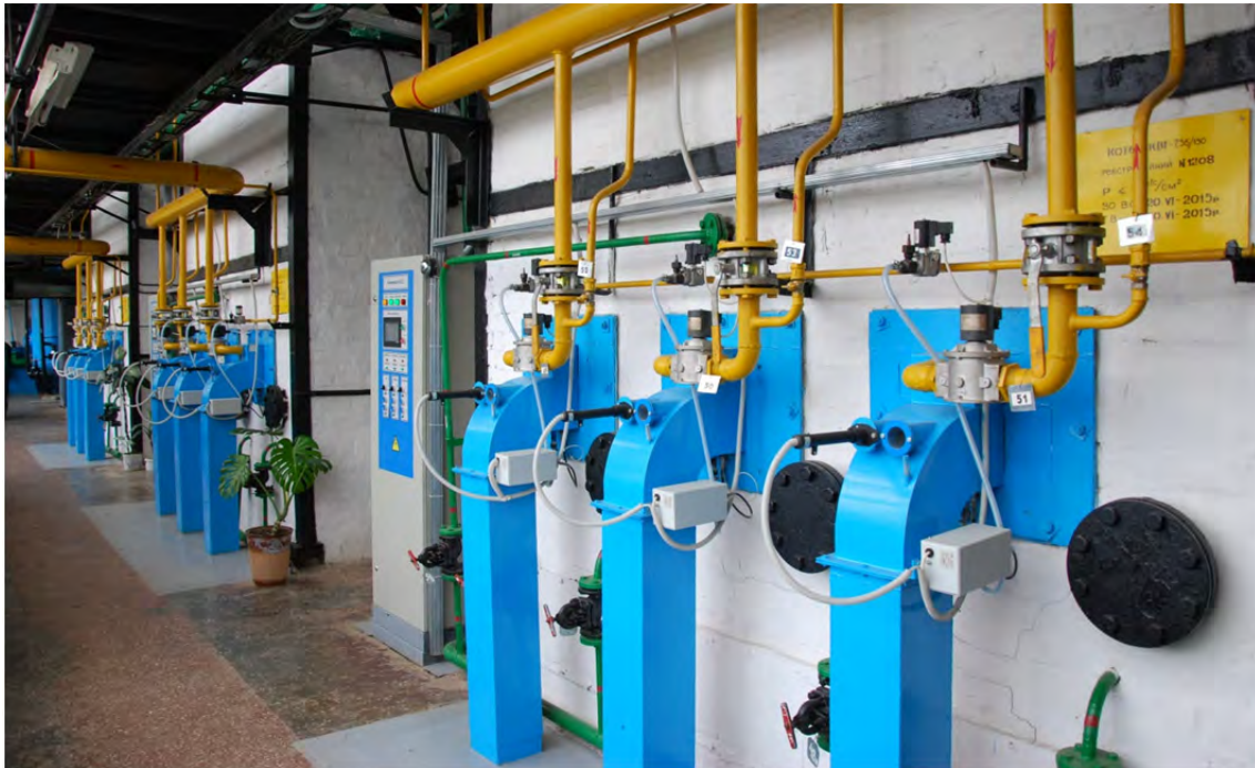
Water-heaters with MD Gas Burners
